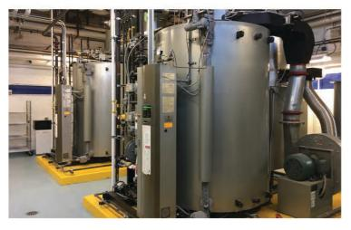
The 'floating header' concept allows for even thermal expansion of the tubes, therefore reducing stress points within the boiler." The 'leaky tube' problems associated with firetube and bent watertube designs have been eliminated. The main mechanical contractor for the UnityPoint Health -Meriter project was AMS Steam Products of Milwaukee, WI, (www.american-boilers.com) a Wholly Owned Subsidiary of Hot Water Products, Inc.
