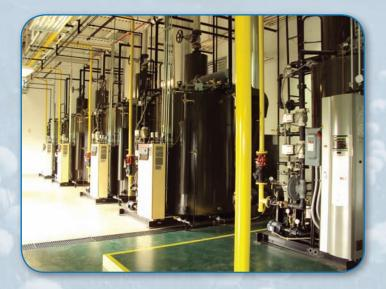
"We're running anywhere from 80 to 87 percent efficient with the Miura boilers. We have an erratic steam load, but you can bring these boilers up fast and have them online in about ten minutes."
