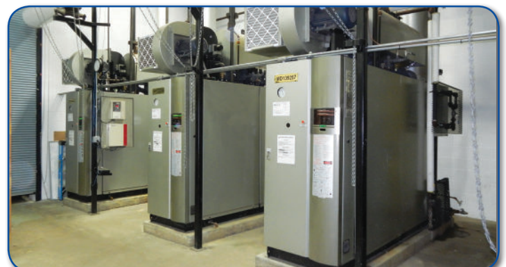
Three Miura LX-200 steam boilers provide efficient operation at Up to Date Laundry.
